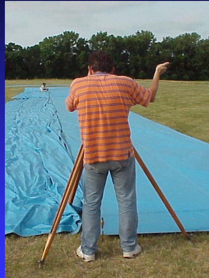
Every stake was aligned by transit.
