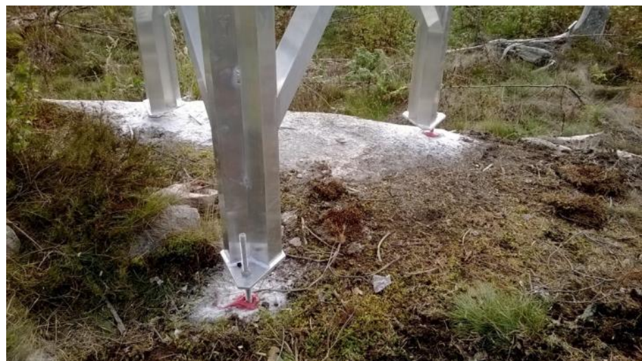
Figure 9: Where applicable, mounting on stable bedrock is a good alternative to a concrete foundation. Example from geodetic observatory Metsähovi , Finland. According to recommendations from the Finnish Geodetic Institute (FGI), the stand of the corner reflector was mounted on the 22mm rods. The holes drilled directly into the bedrock (~40 cm deep) were filled with rock epoxy glue manufactured by Hilti . (© images by FGI)
